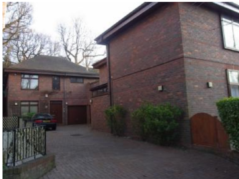
No. 17 (foreground) and No. 16 (background)
