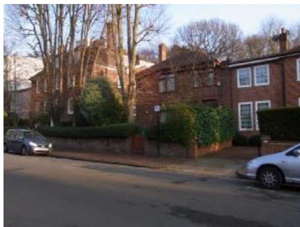
Street elevation of No.17
