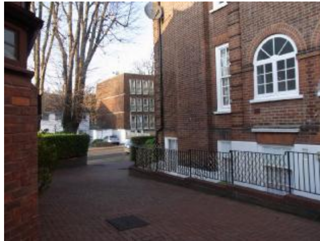
Relationship of the driveway / hardstanding area with the lightwell to the adjacent property
