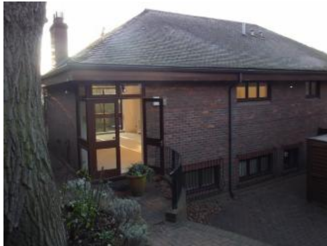
First floor living room of No.16 viewed from the rear garden
