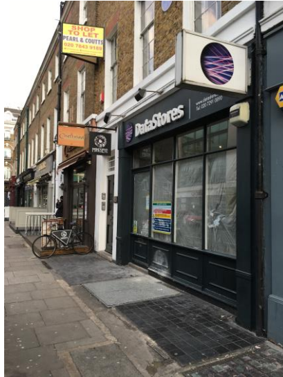
Oblique View of Street Frontage
