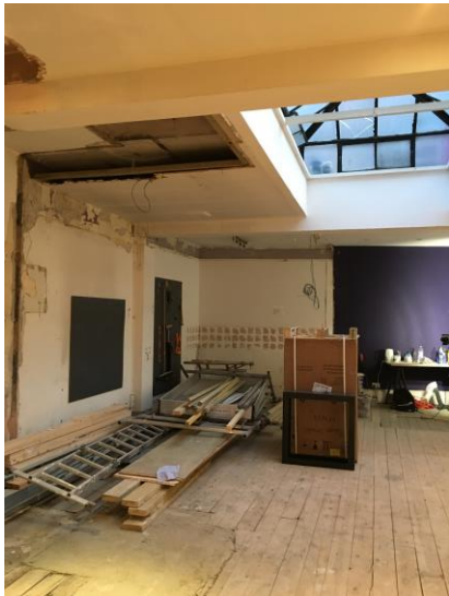
View of interior at ground floor level
