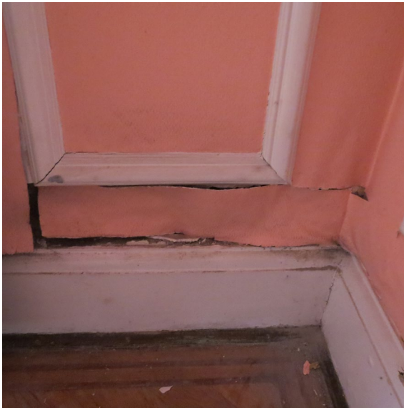
fig 5 & 6. Internal damage caused by damp, ground floor
