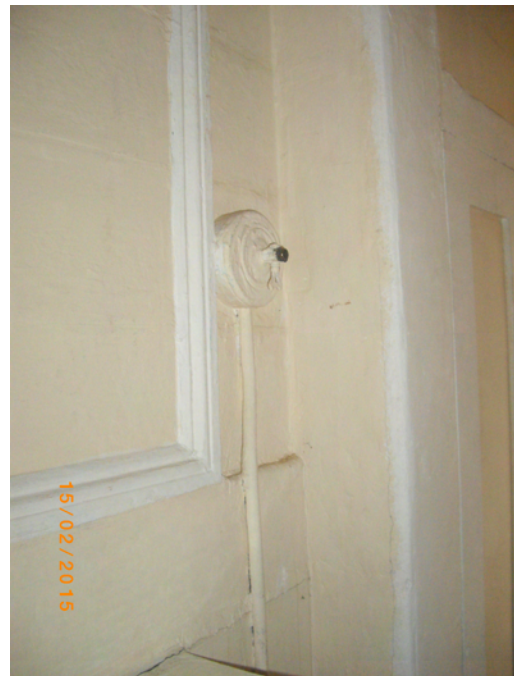
Gas supply for gas lighting, 1 st Flr.
