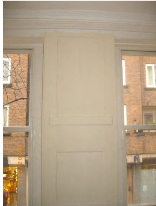
Original panelling between Victorian Vertically sliding sash windows.
