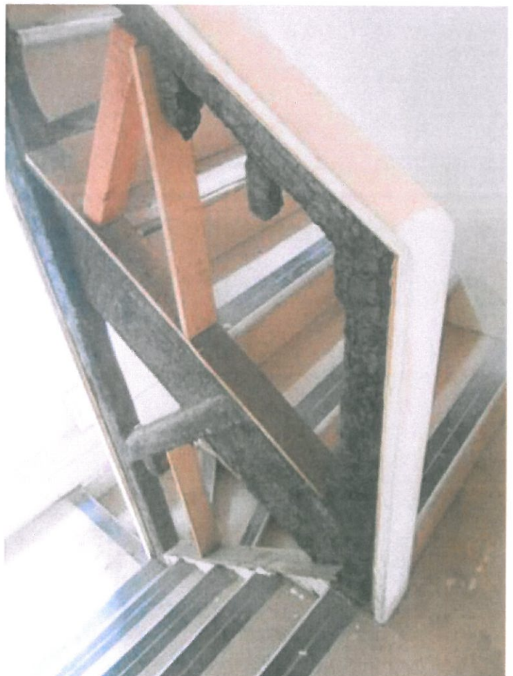
Upper stair flight showing burnt oak stair spindles and charred newel post and stringer
