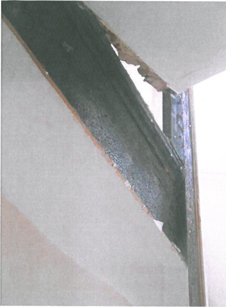
Upper stringer and newell post with light surface charring
