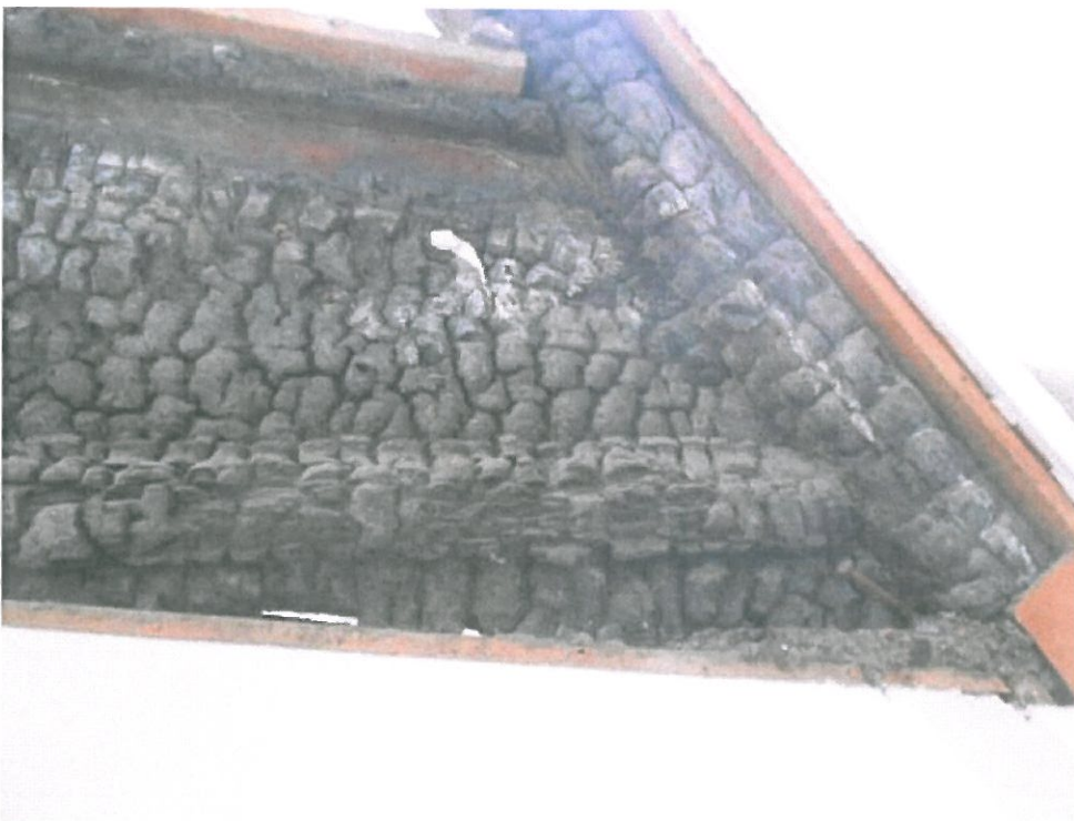
Extensive charring at stringer to newell post junction
