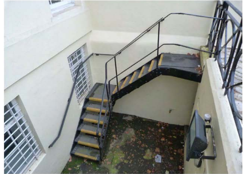
Northern lightwell with modern metal steps
