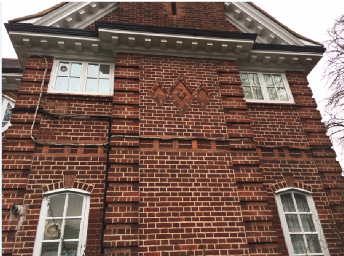
Right hand side of front elevation - original windows at ground floor and replacement windows at first floor
