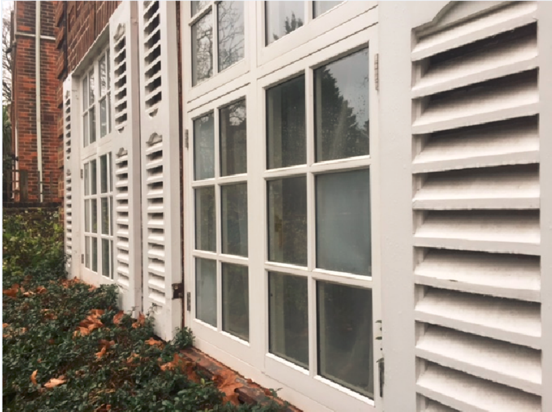
Close up of ground floor front elevation replacement windows
