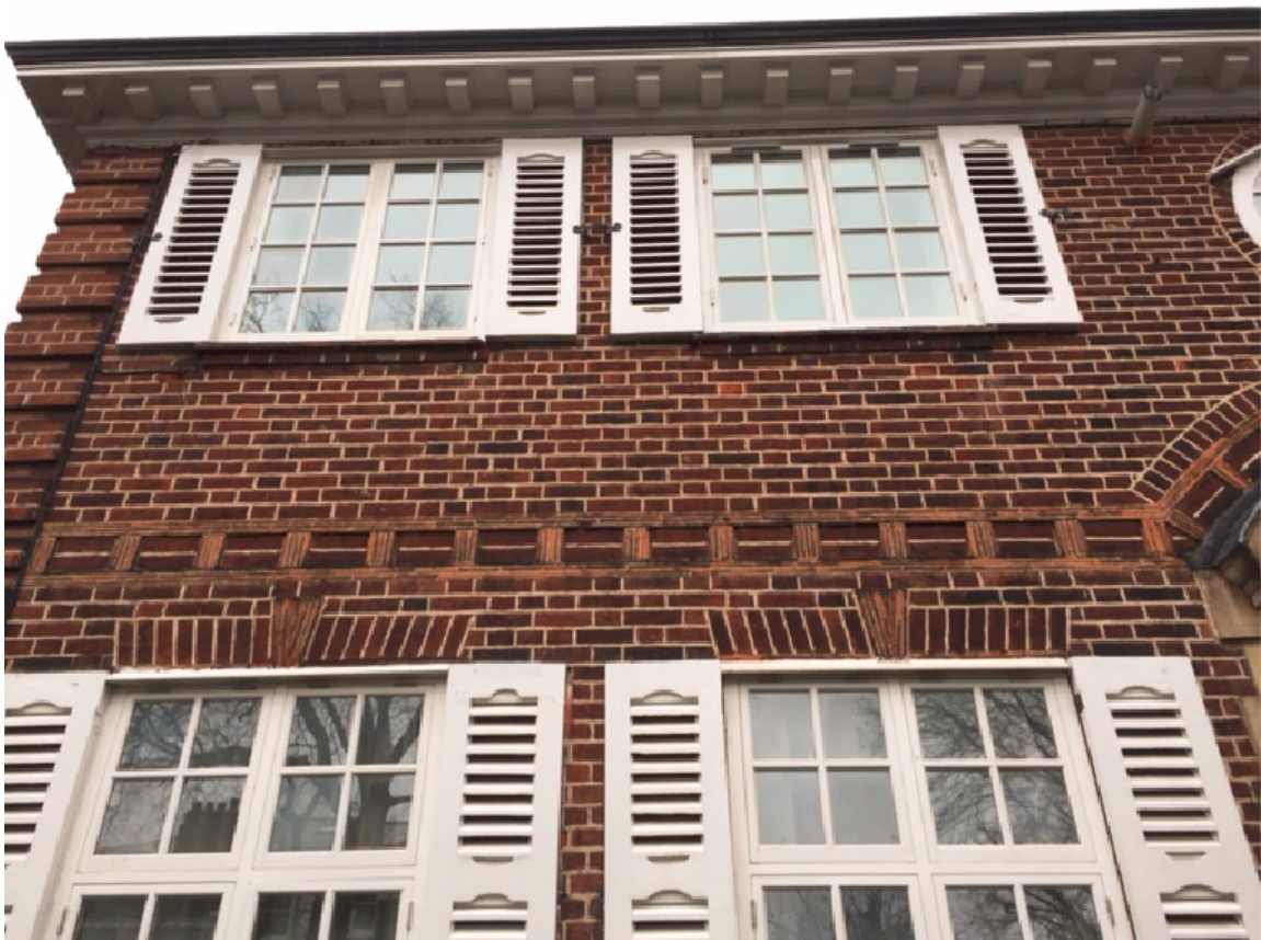
Left hand side of front elevation showing 4 replacement windows
