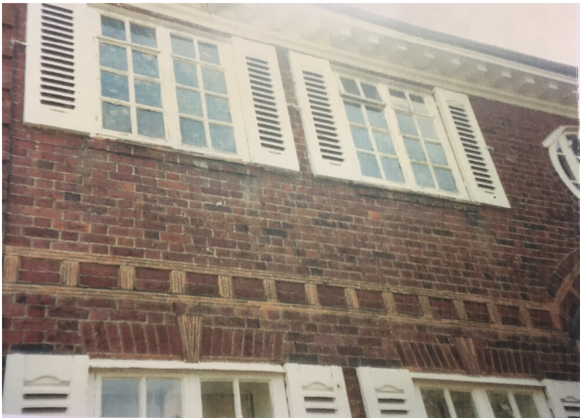
Original windows to front elevation
