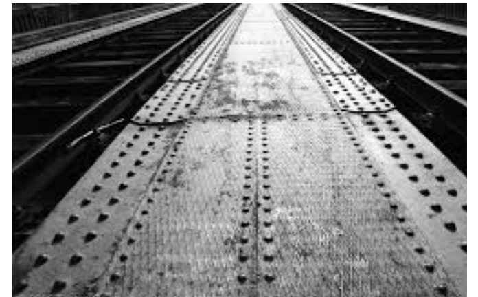
Riveted 'railway' metalwork
