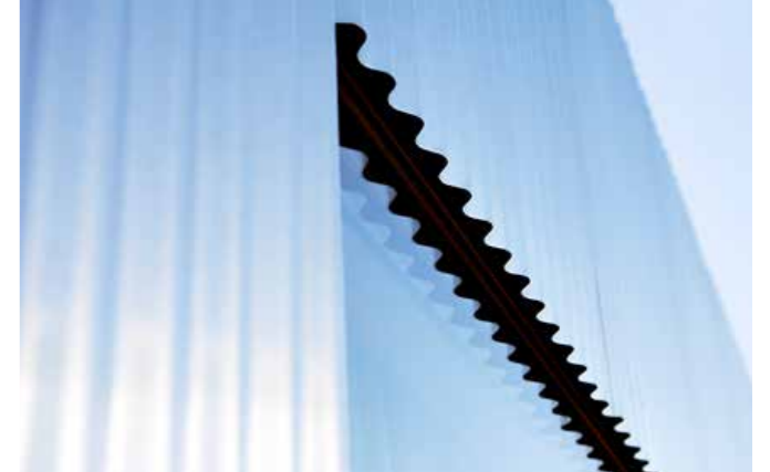
Carefully detailed corrugated metal cladding
