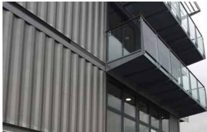
Dark grey metal of the 2015 Container Building
