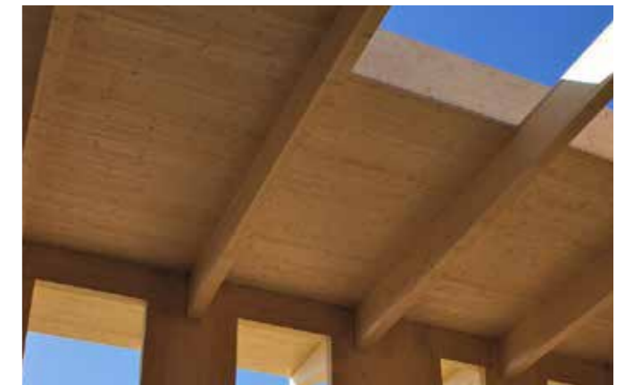
The CLT structure will be exposed in Studio C
