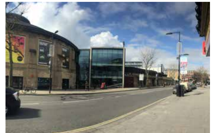
Existing condition with dilapidated fencing and advertisement billboards
