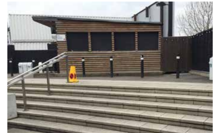
View of existing Tiki bar from bottom of steps
