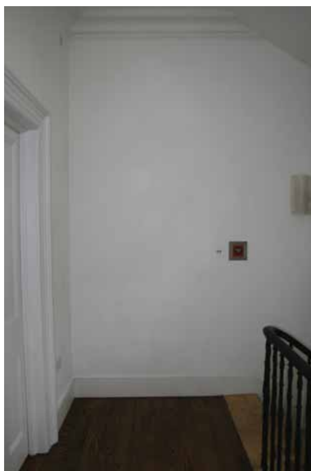
3.19: First floor landing (position of former door)
