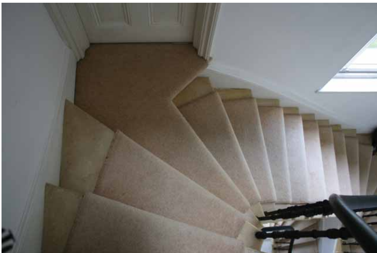
3.26: Second floor stairs
