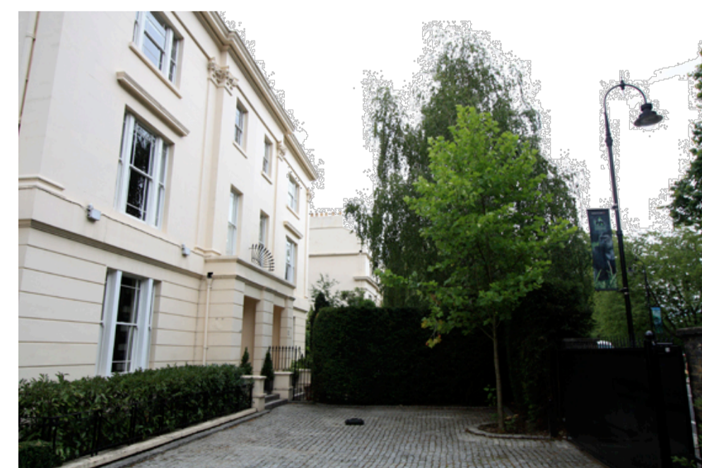
Front Drive Way - Looking East
