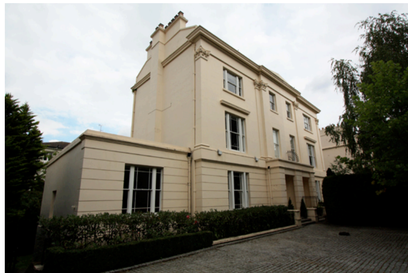
13 Prince Albert Road - Front elevation
