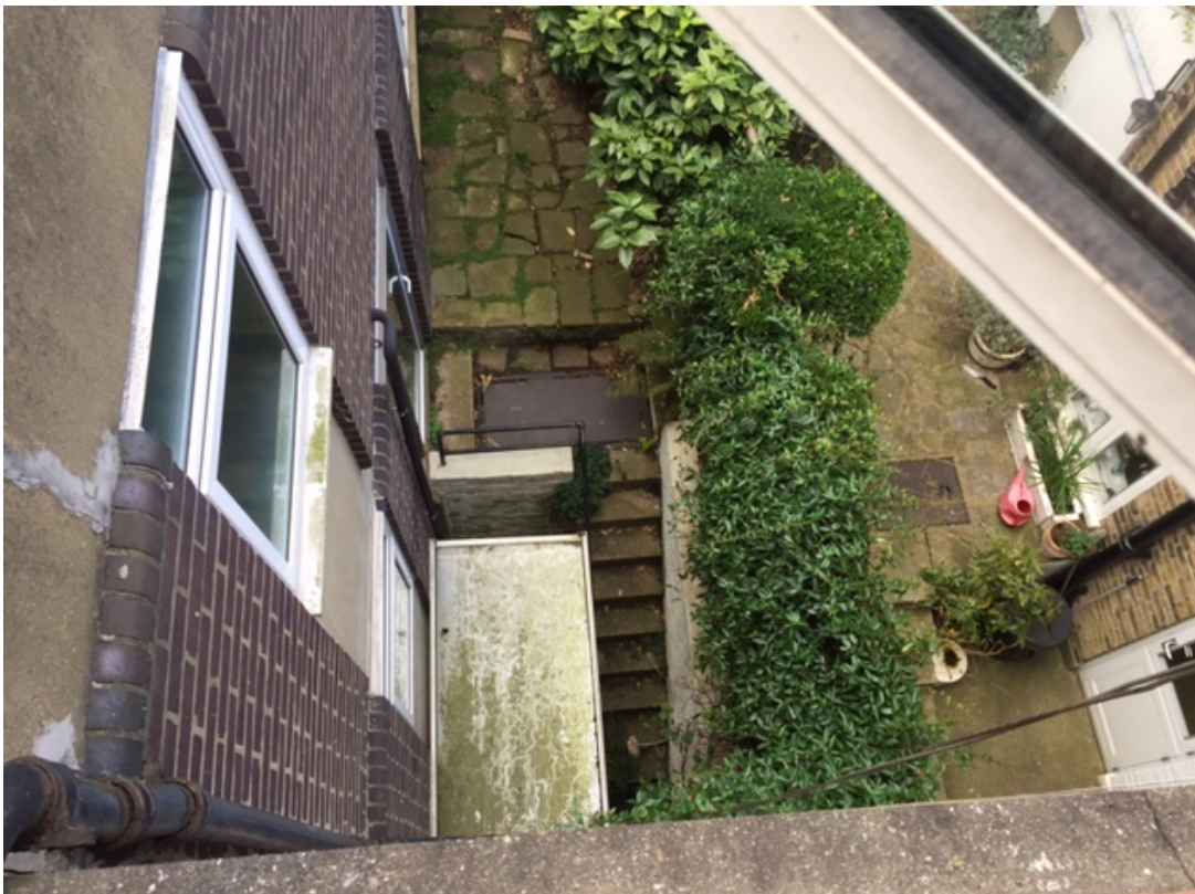
Photo 8: View from 2 nd floor window of existing lightwell
