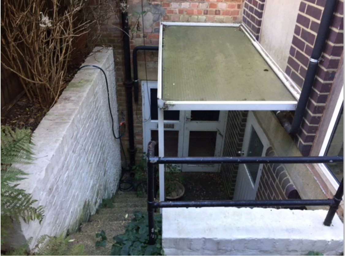
Photo 9: External view of lower ground floor lightwell area
