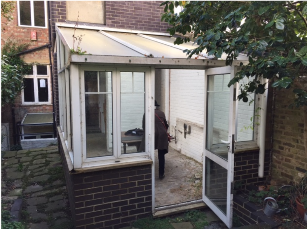
Photo 5: Existing single storey conservatory
