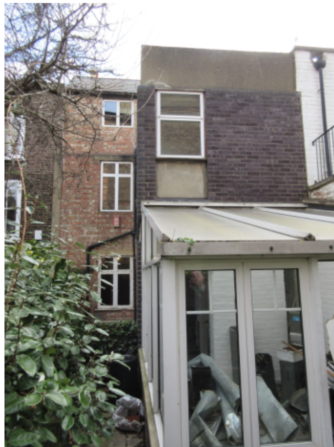
Photo 6: Existing 2 storey rear extension and rear elevation
