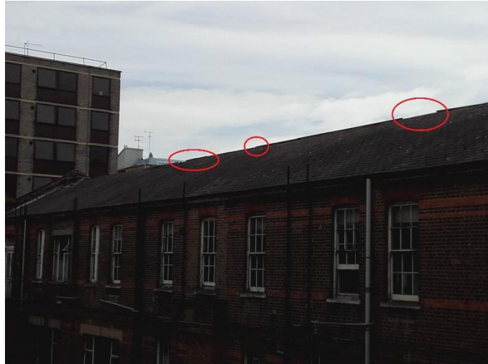
Photograph 8 Missing / lifted ridge tiles on B3.2
