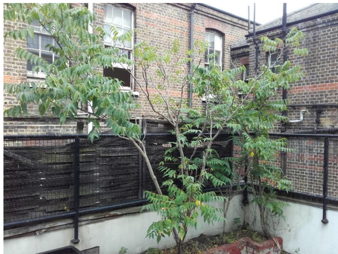
Photograph 2 Flat roof section of B2 with ash saplings growing through
