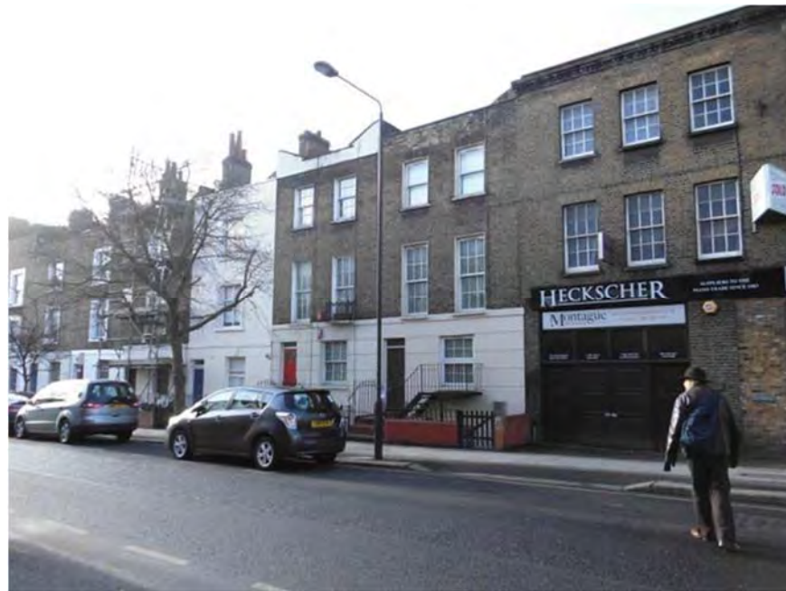
Photograph 6 – View of front of the building
