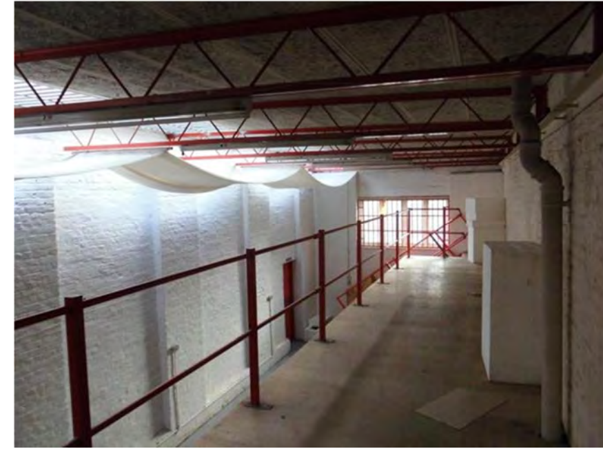
Photograph 7- Internal view of rear 'leg' of building
