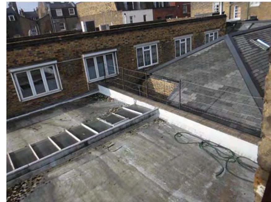
Photograph 8 – View from front building of lower roofs
