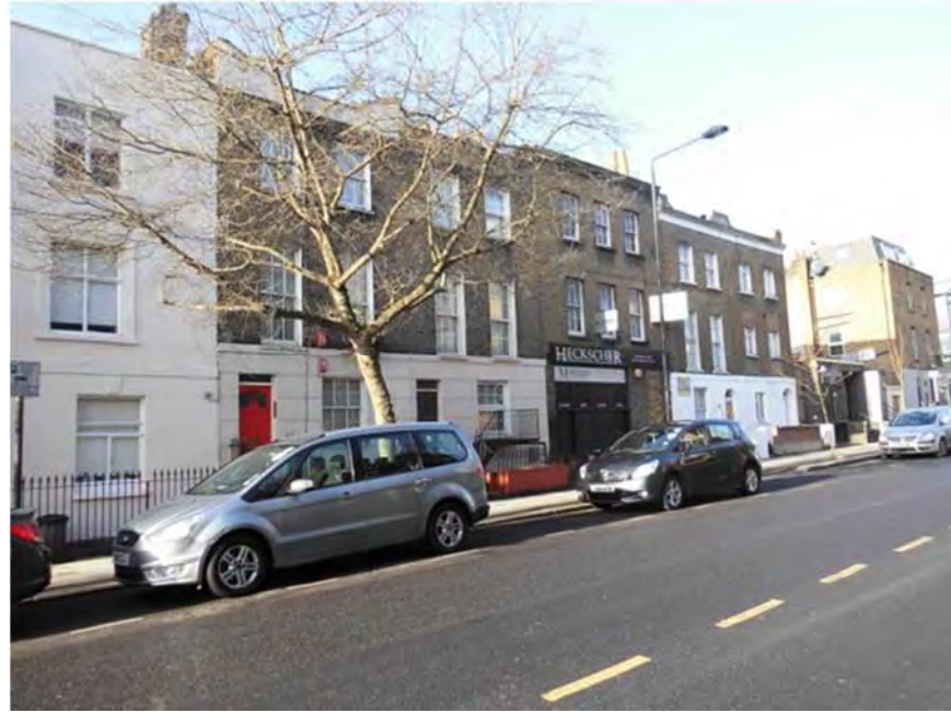
Photograph 5- View of front of the building
