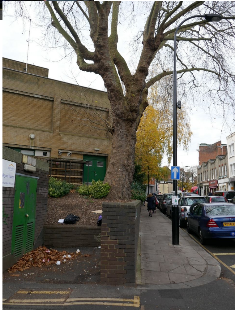
2) View along the wall showing lean in the wall and the tree's trunk and the crown overhang which would impede piling equipment.
