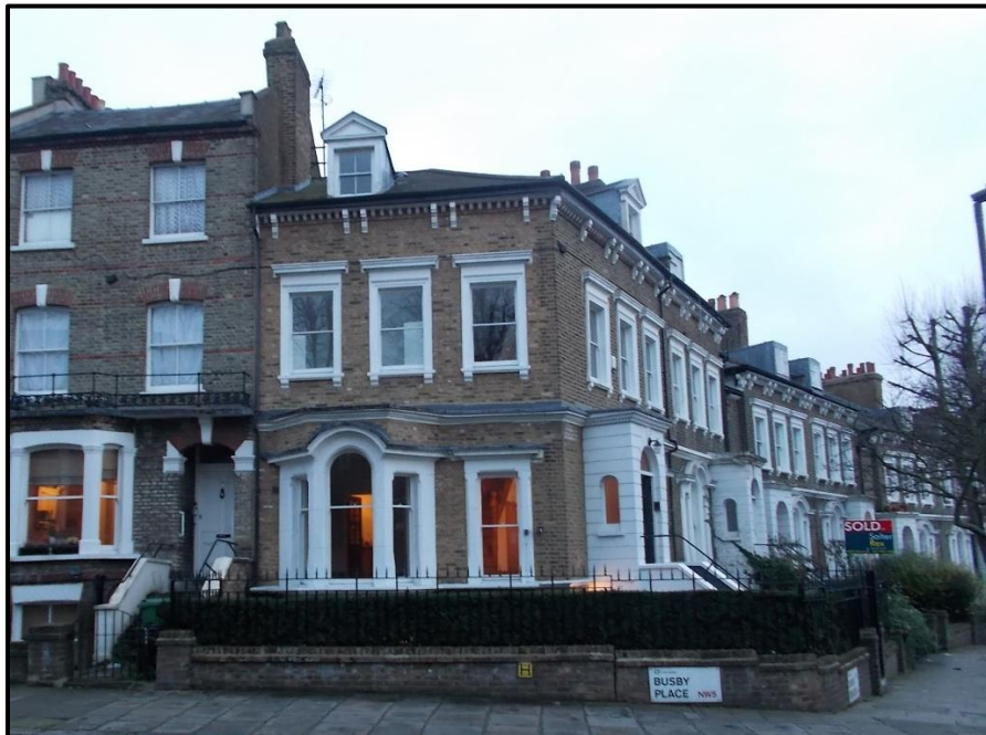
Fig. 3: Secondary front elevation 32 Oseney Crescent
