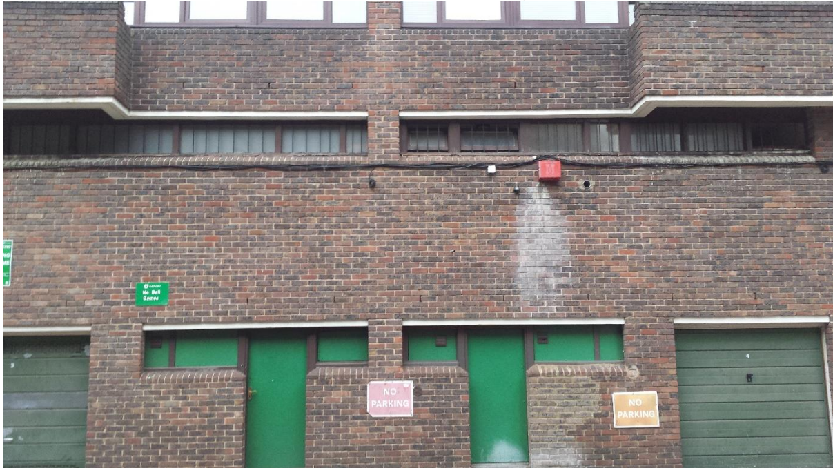
Rear of Site (from 1metre outside Flat No.6 Fordcombe House)
