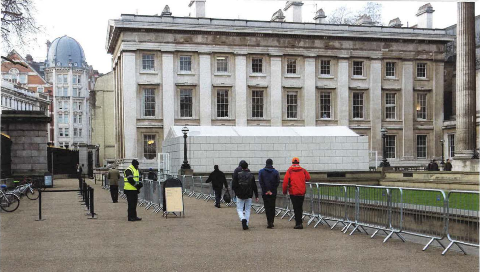
South Security Structure
