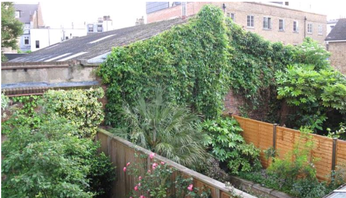
View showing the pitched section of the building behind Nos 5 and 6 Collard Place
