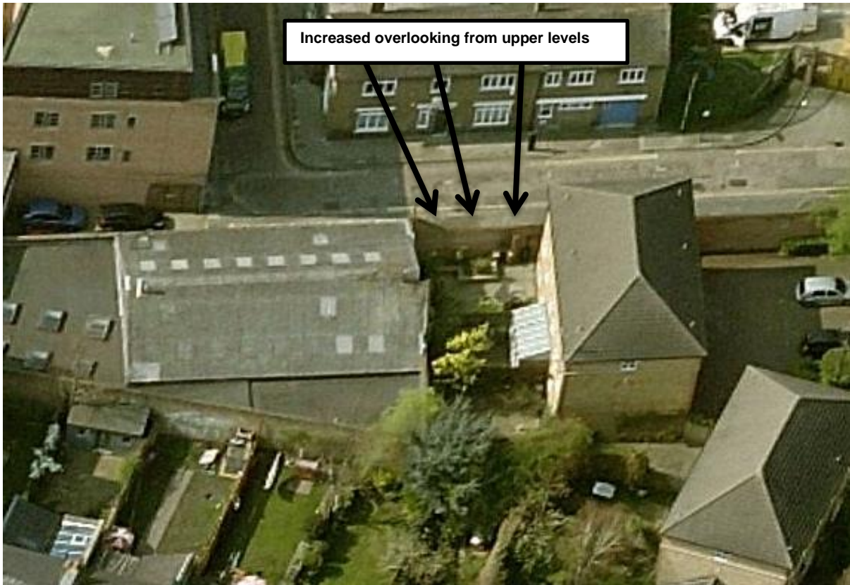
Aerial photograph demonstrating addition overlooking from proposed site B
