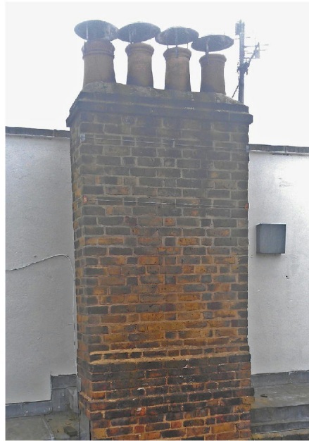
fig 8. Chimney stack extended by works at No. 36
