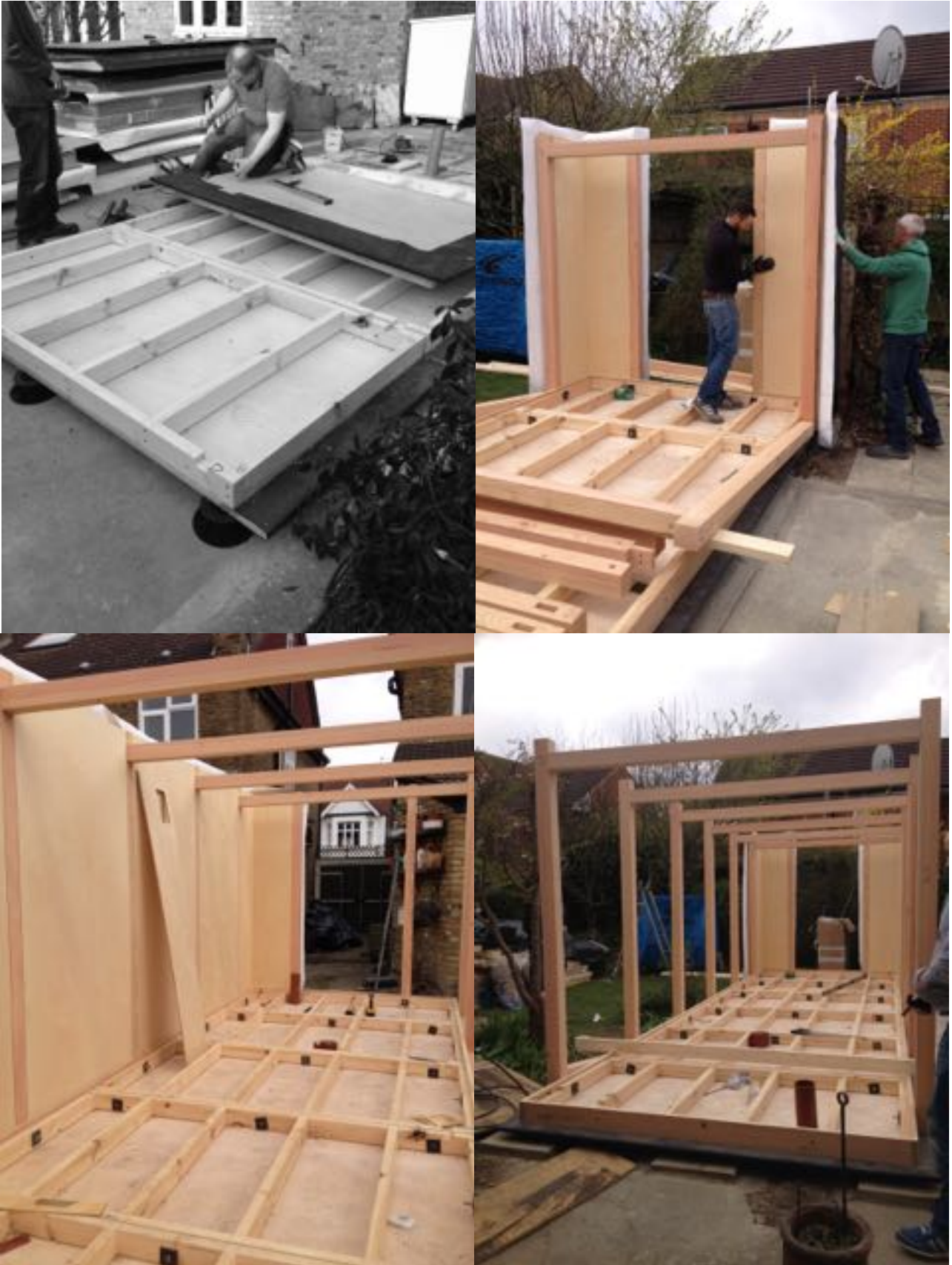
fig2: 3rdSpace under construction
