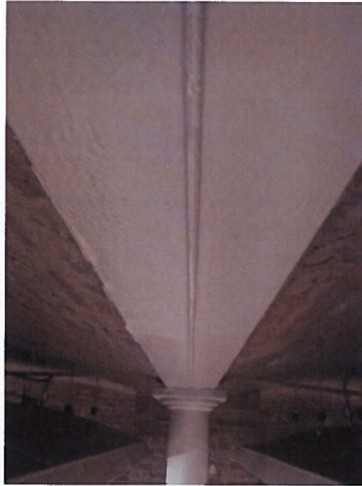
Photograph 5. Showing a length of the wrought iron beam
