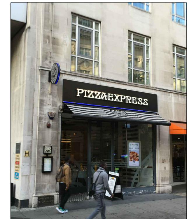
EXISTING FASCIADE PHOTO
