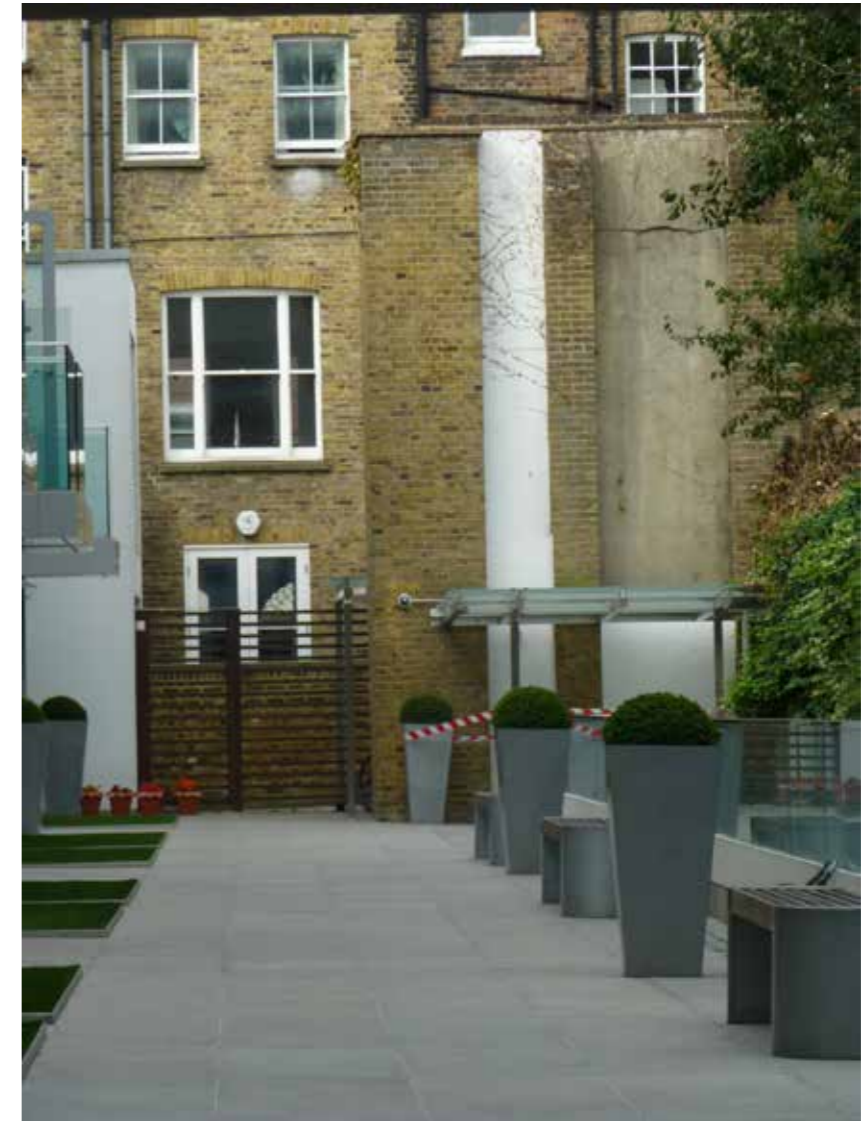
Image 9: Rear wall from 7-15 Whitfield Street
