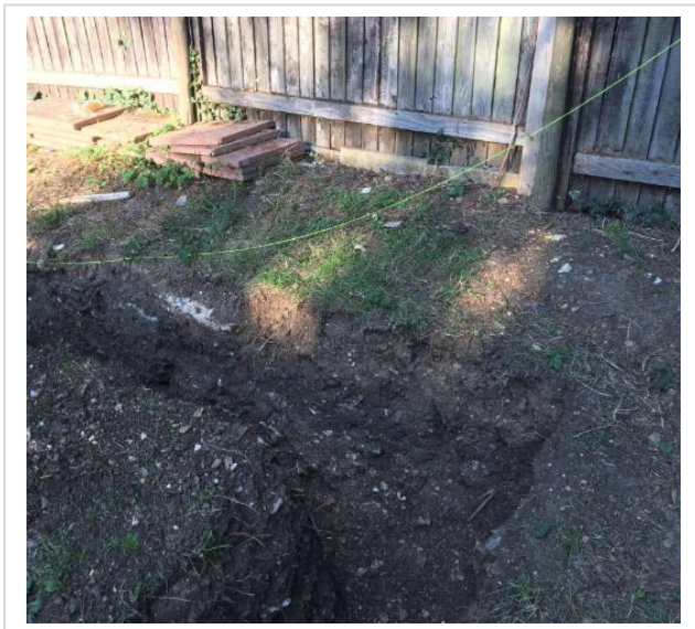
Example of hand-dug trench
