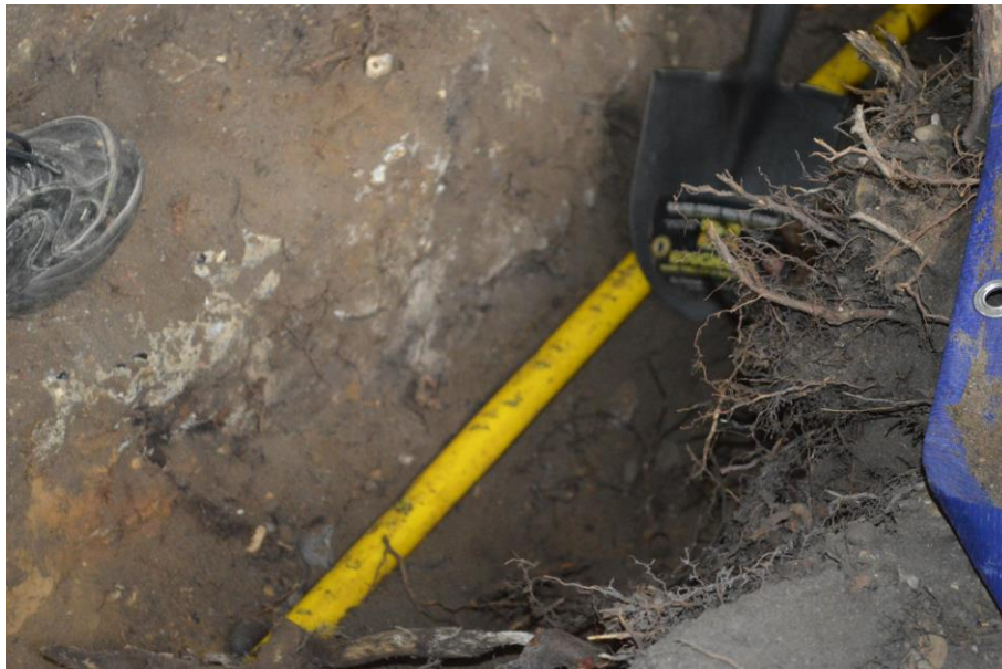
Photograph 4 Gas pipe running alongside the garage wall.
