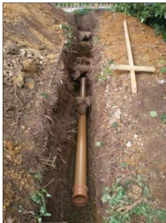
Services image 2: Continuous trenches dug by hand so that important roots can be retained (with the service ducting threaded beneath) is an effective means of minimising damage (note the ground protection boards with soil piled on top on the left).
