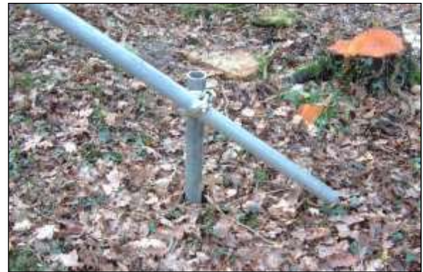
Fencing image 3: Close up of bracing detail, essential for increasing the stability of the vertical framework.
