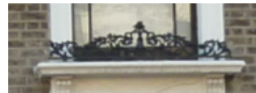
existing cast iron window box retainer to front of 6 Princess Road
