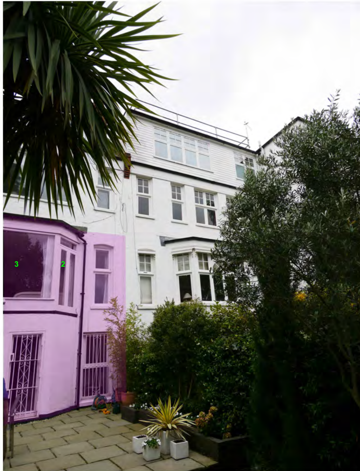
1 VIEW TO NORTH EAST (STUDIO FLAT & FLAT No 3 TERRACE)
