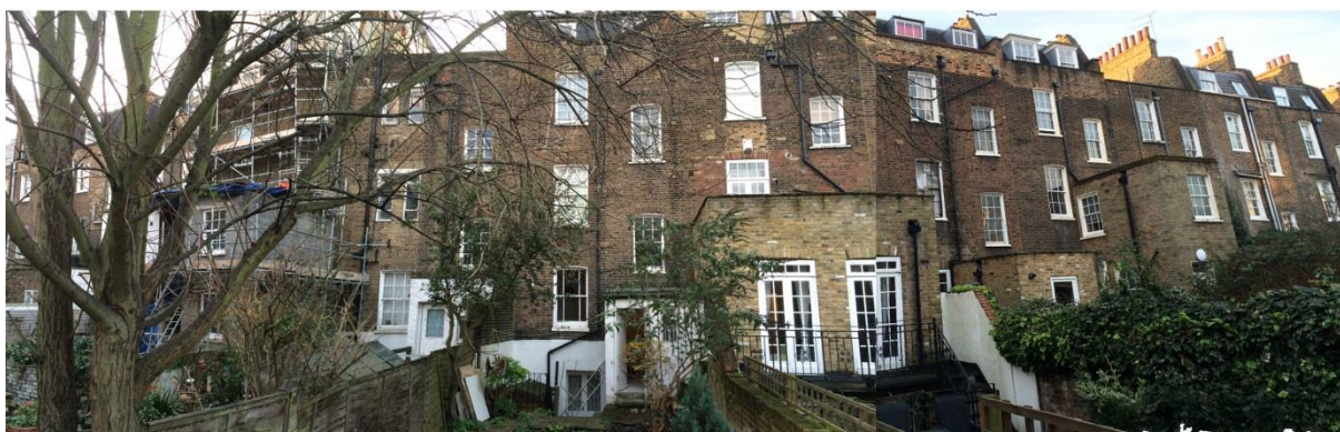
Photograph of rear elevation from garden level (Photograph taken January 2016)
