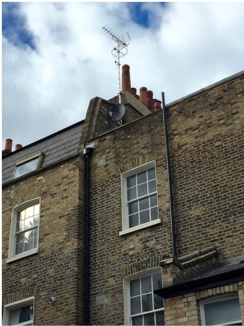
EXAMPLE OF IRS INSTALLATION - SATELLITE DISH (PAINTED BLACK), TV & RADIO AERIALS (at 33 FREDERICK STREET)
