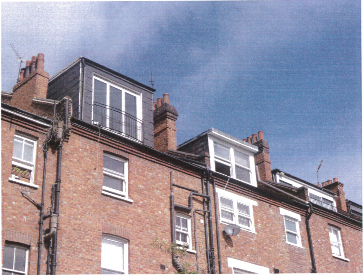
Photo 10. Adjoining dormers to the north east in the Terrace
