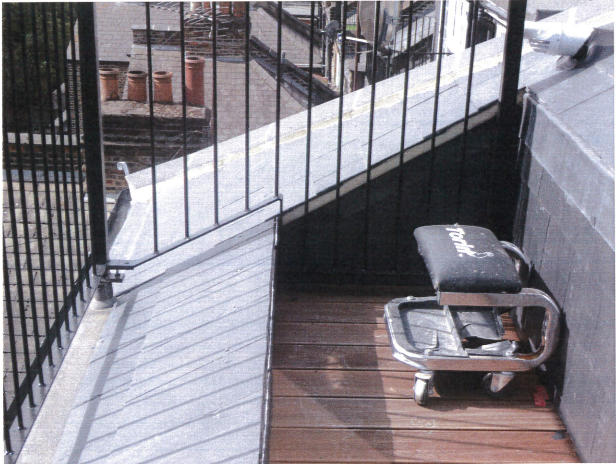
Photo 7. View inside the terrace of the rear dormer.
