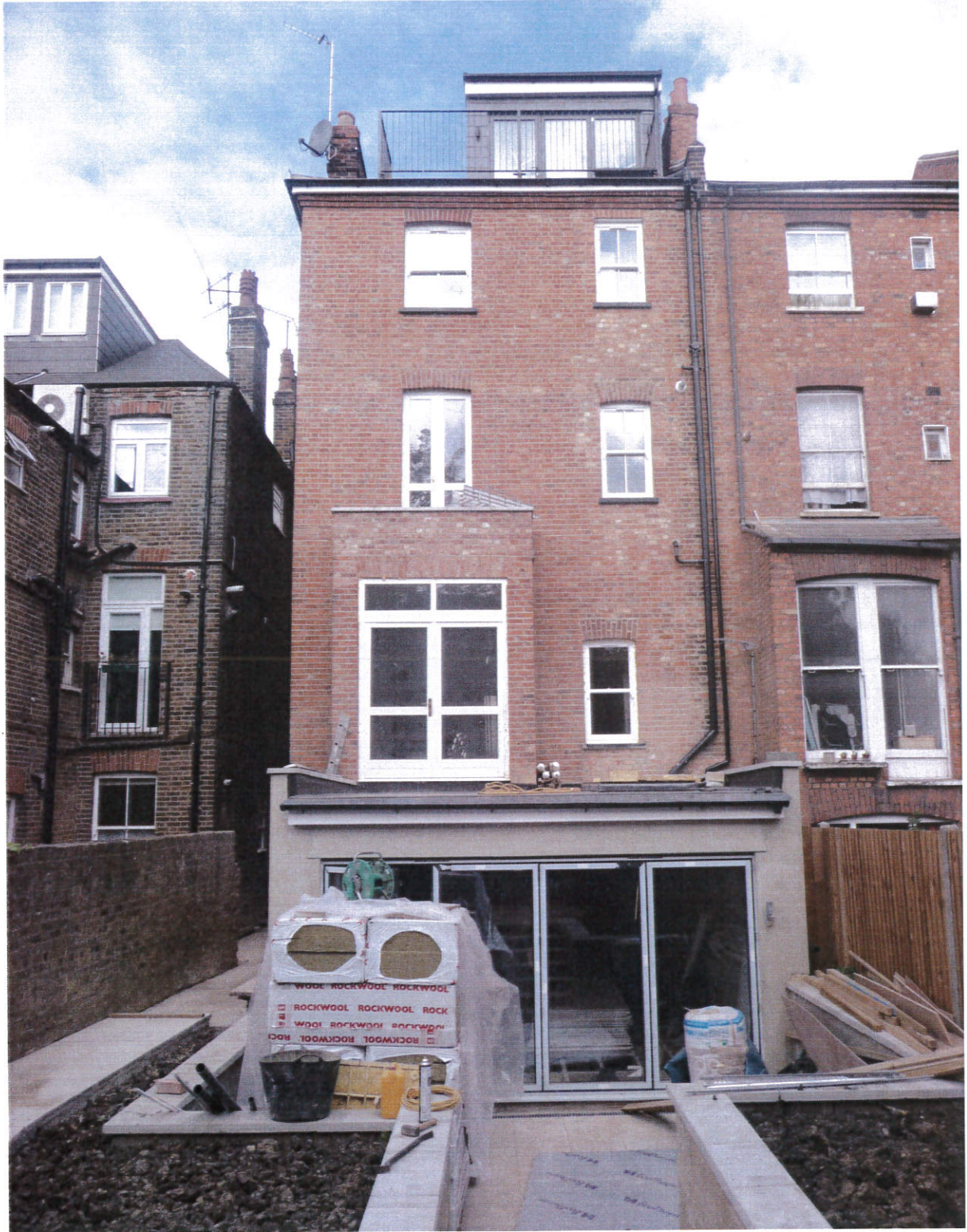
Photo 5. Rear elevation under construction.
