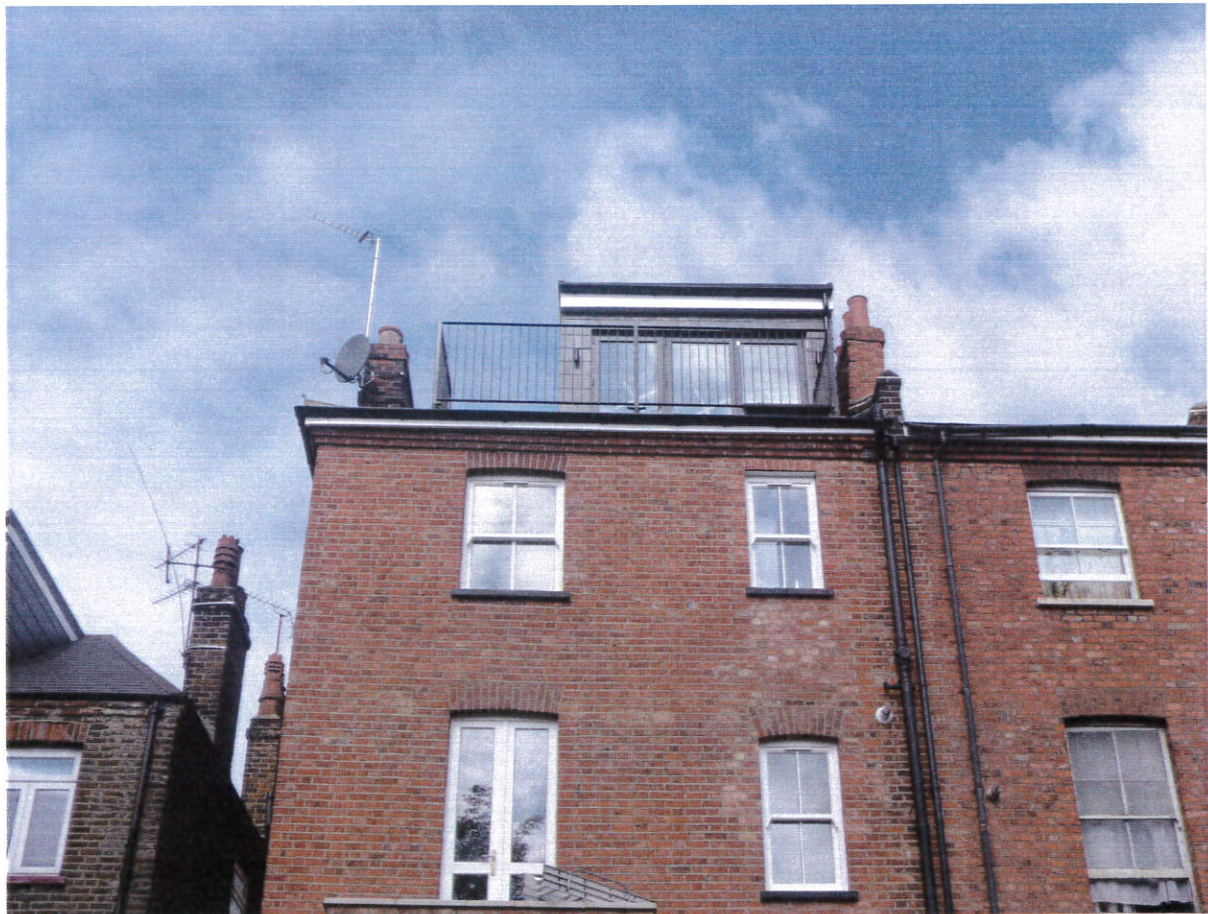
Photo 6. The rear dormer as constructed.
