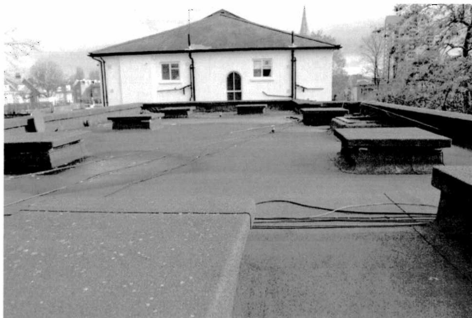
Roof of Block 7-12 standing west looking east
