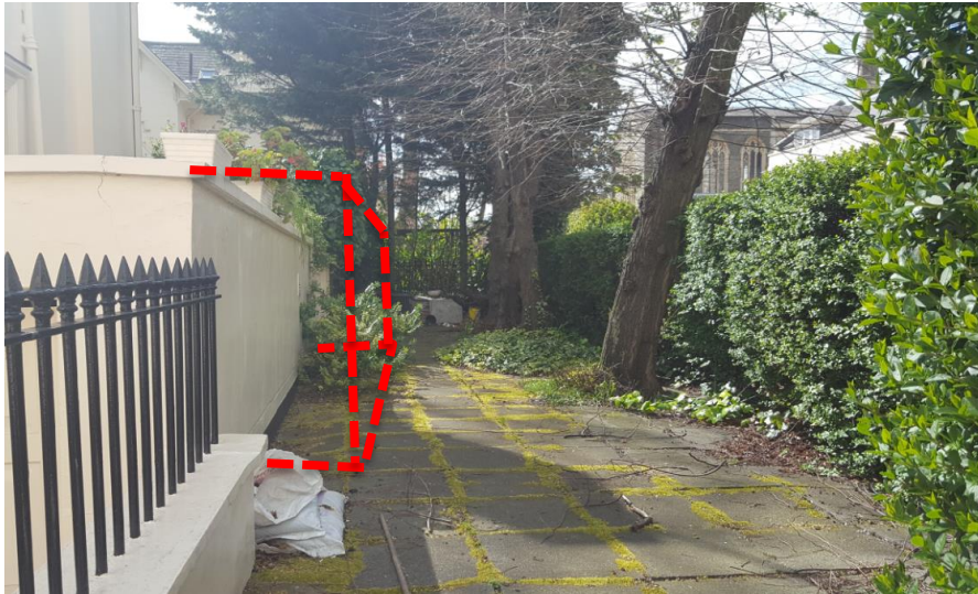
View along the side of the garage showing previously permitted extension dashed in red
