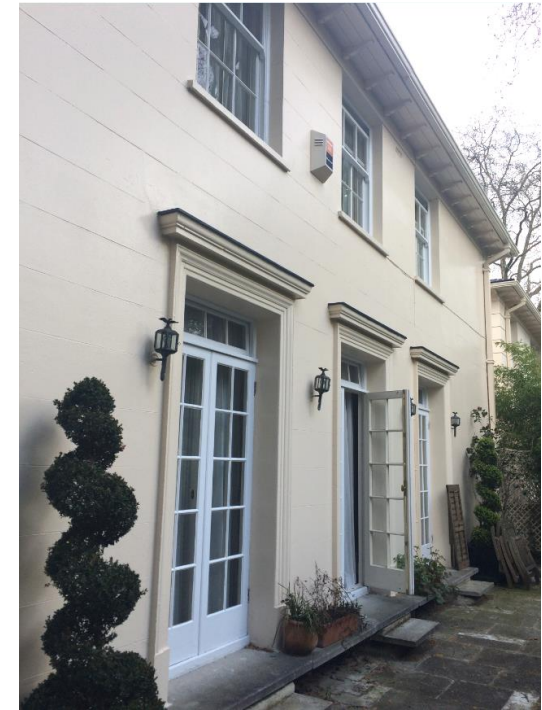
View of the rear elevation
