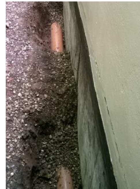
Trial trench photograph
