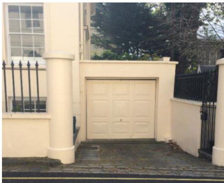
Frontage of existing garage
