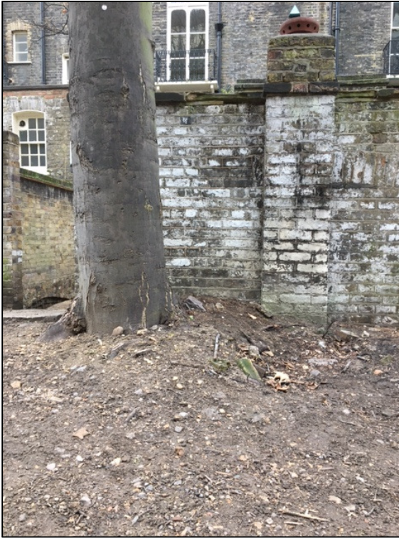
Figure 2: Soil heave indicating presence of large roots
