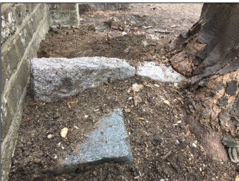
Figure C: Bricks being pushed towards wall
