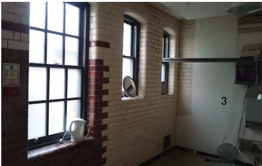
Existing ground floor (rear)
