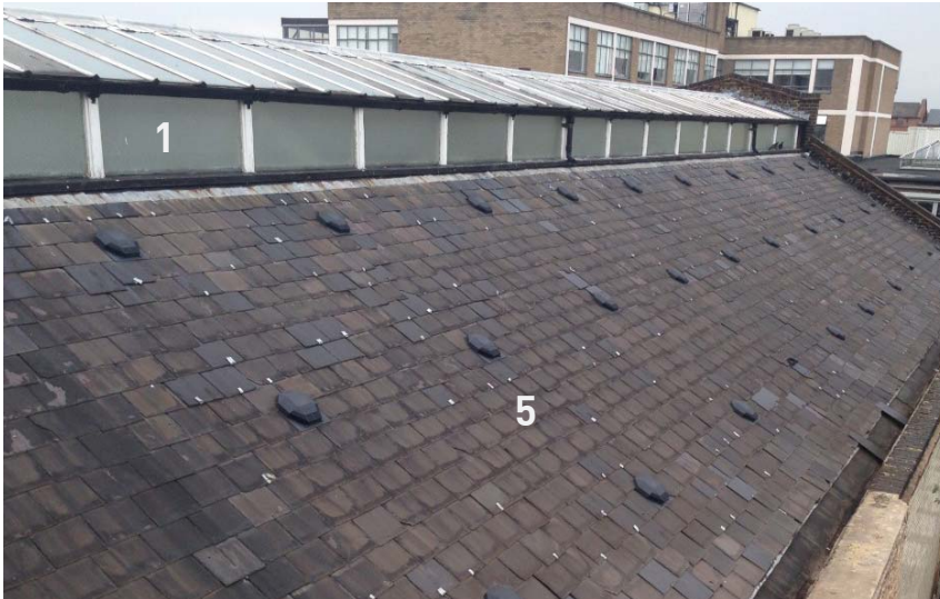
Current slate roof covering
