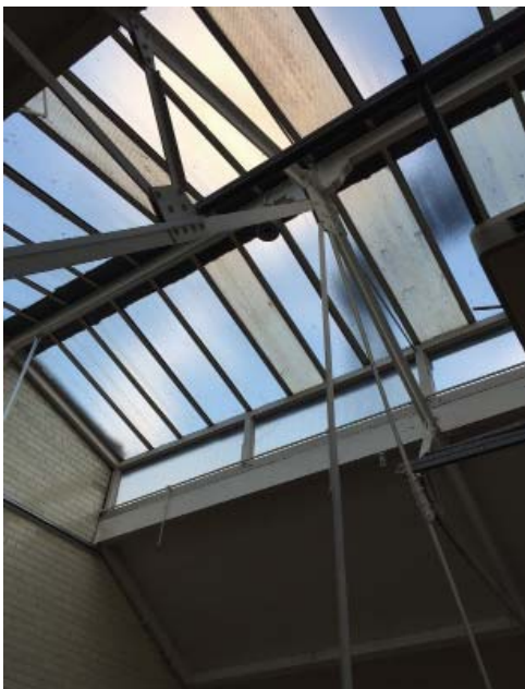
glazed roof lights
