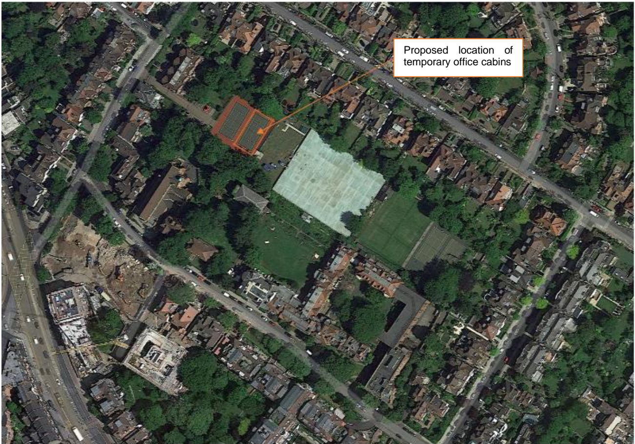
Aerial view of the site with indicative cabin location highlighted by the orange line.
