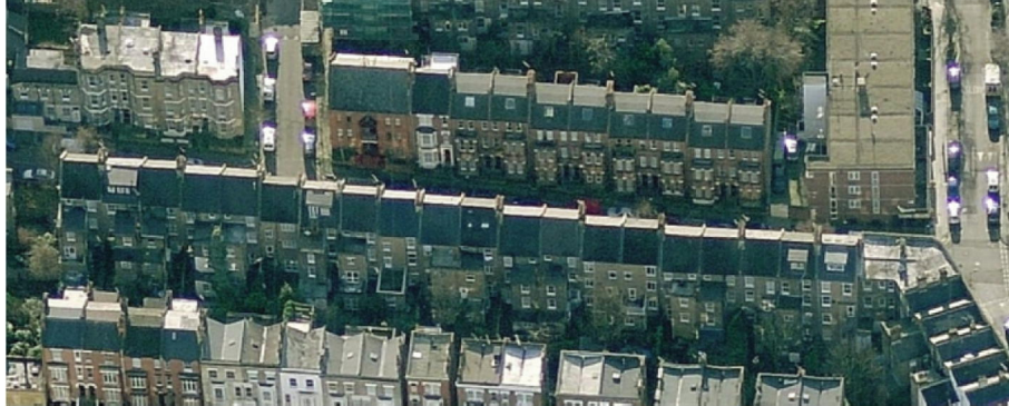
Figure 1 - The roofscape along Gascony Avenue
