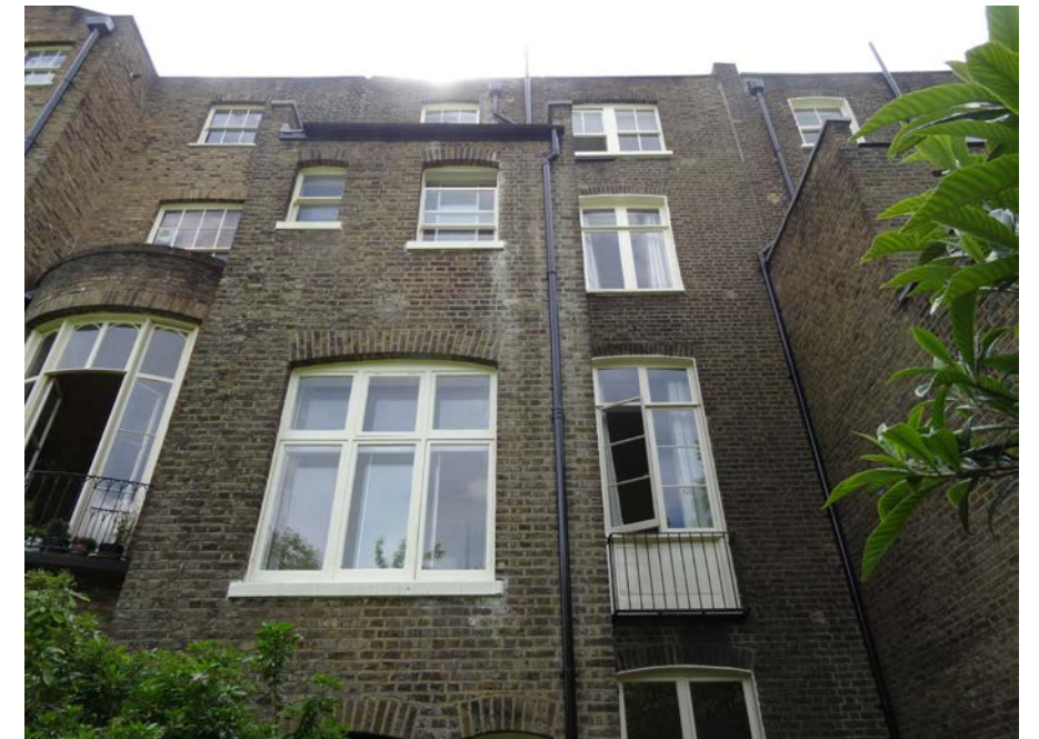
View from Rear Terrace of Rear Elevation
