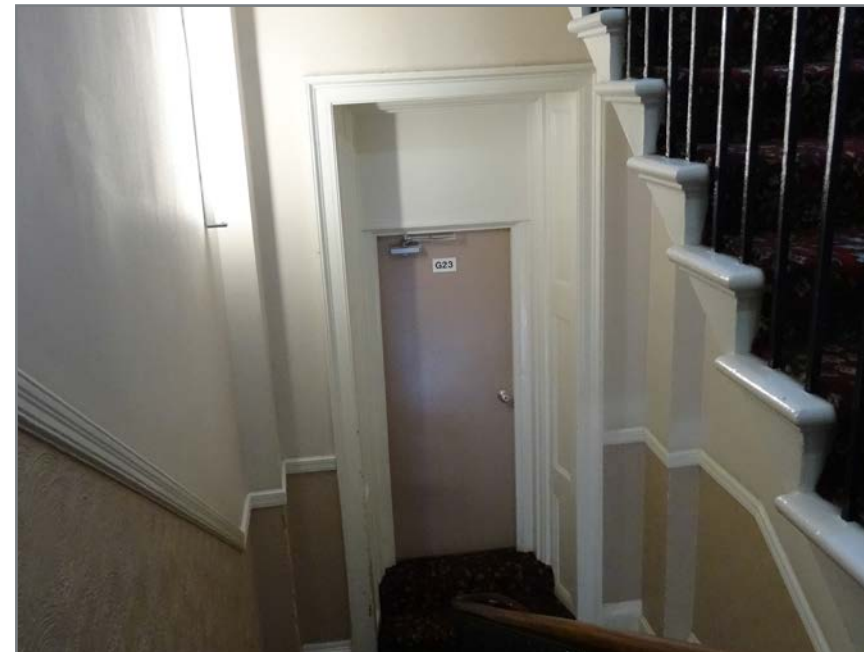
Architrave and Panelling to Door at Half-Landing
