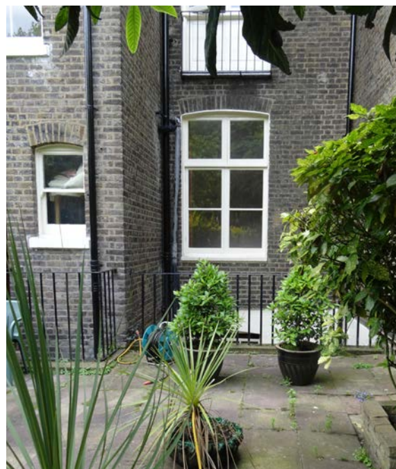
Rear elevation of 24 Montague Street
