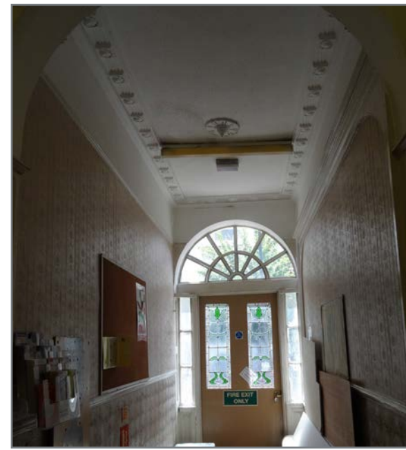
View of Entrance Door and Fanlight
