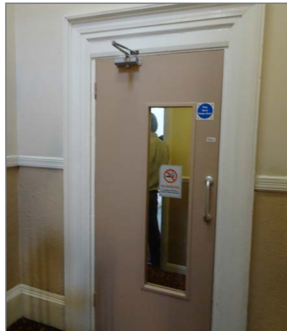
Original Architraves and Skirting
