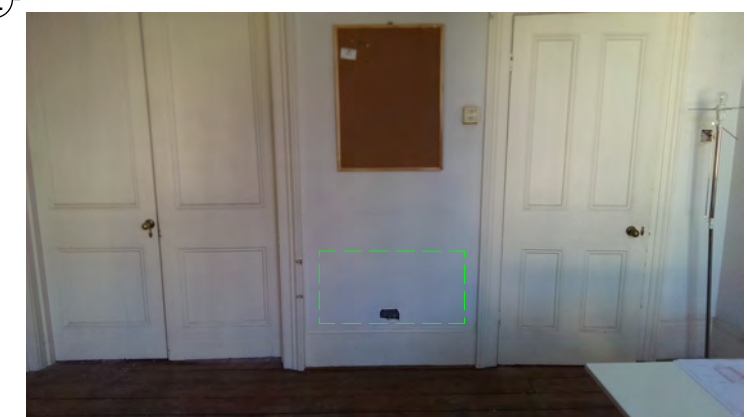
Proposed new radiator location to work best with the existing M&E configuration and BTU requirements. Existing plain wall. New notches may be required in joist for new rad pipes.
