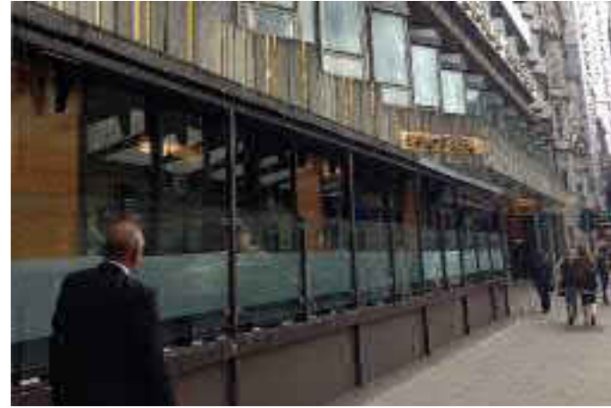
The Imperial Hotel, External Seating Area
