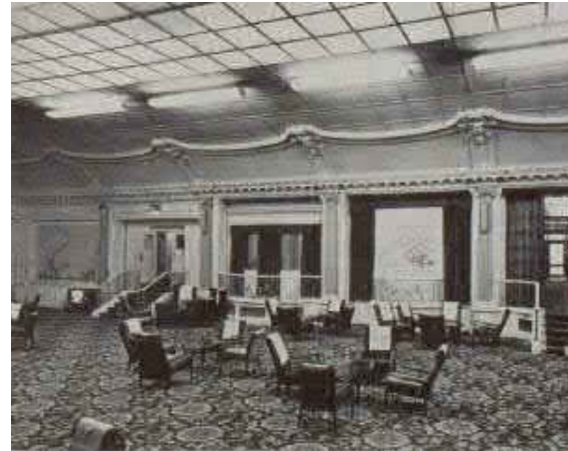
Sunken glass-roofed Winter Garden serving as a lounge to the ballroom. Interior Design Journal 1972
