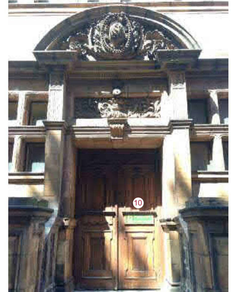
Existing sign 10 - Fire Exit Keep Clear Sign
