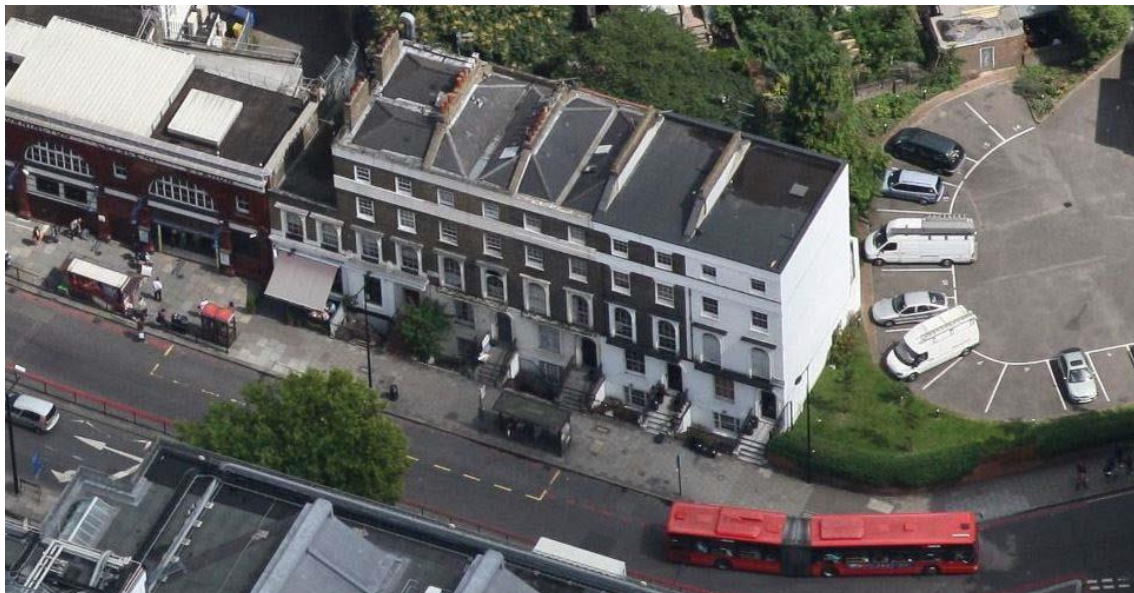
Fig. 3. – Photograph depicting Bus Stop, Bus Shelter, shared-use Parking Bay, Adjacent land car Park.
