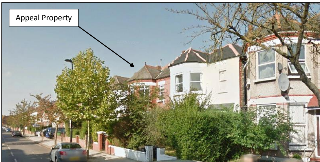
Appeal Property Viewed from the Southeast
