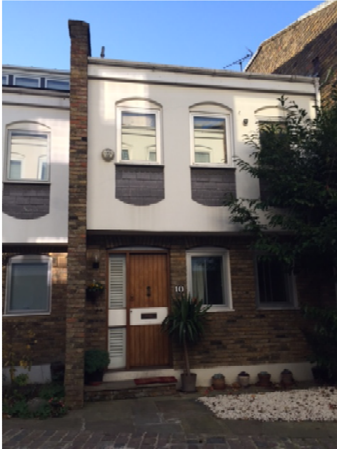
Photo 1 (above): Front elevation 10 Old Brewery Mews
