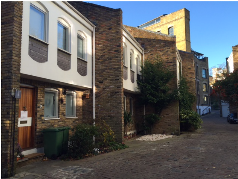
Photo 4 (above): Front elevations of 9, 10 and 11 Old Brewery Mews looking west
