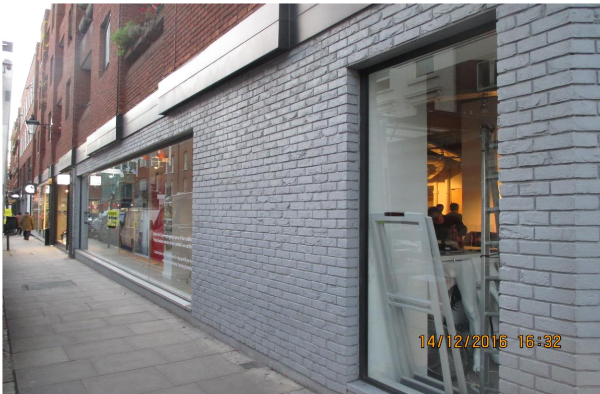
2. Shopfront – showing Earlham Street elevation (existing)
