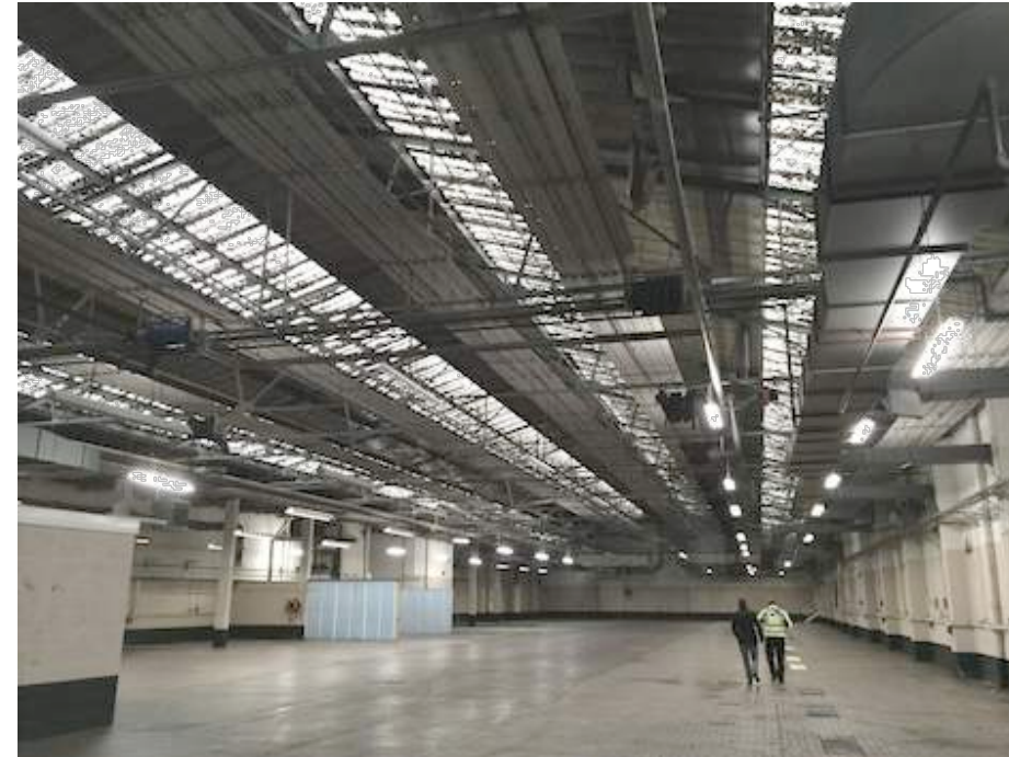
Interior of the existing building
