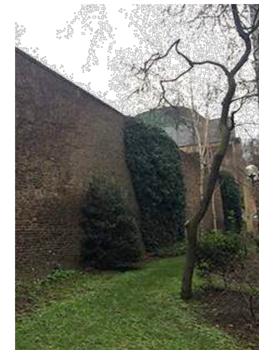
West Elevation - from Birkenhead Estate
