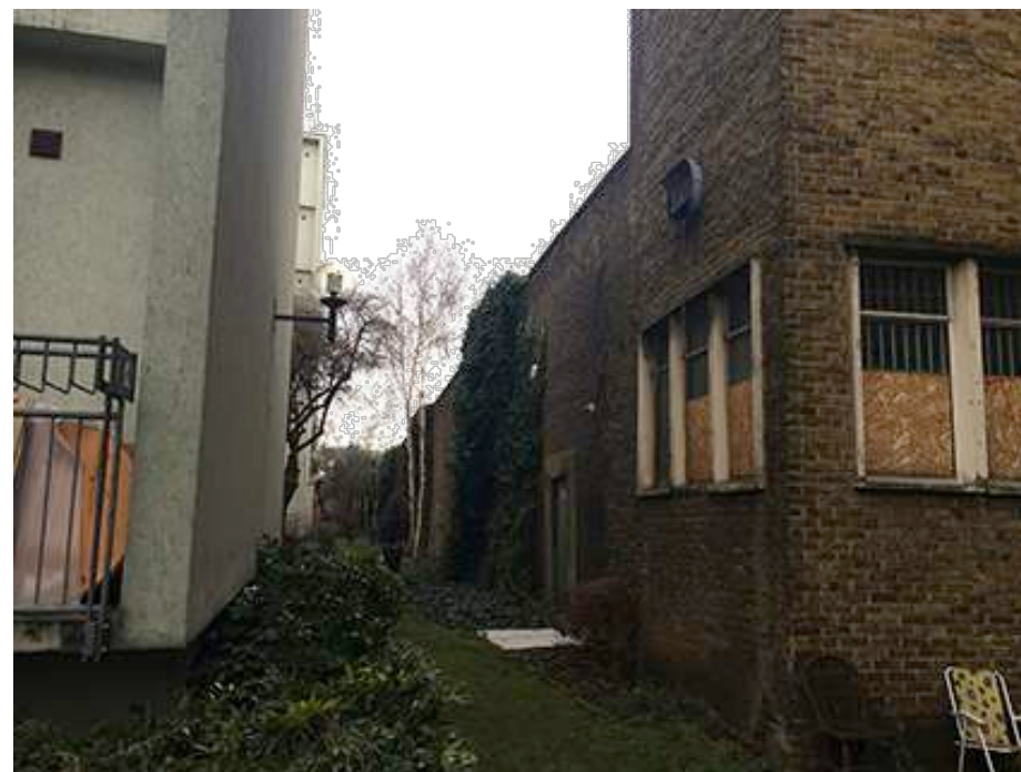
West Elevation - from Birkenhead Estate
