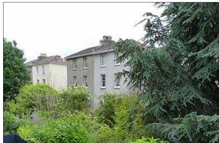
Roof Terraces - raised planters and timber decking
