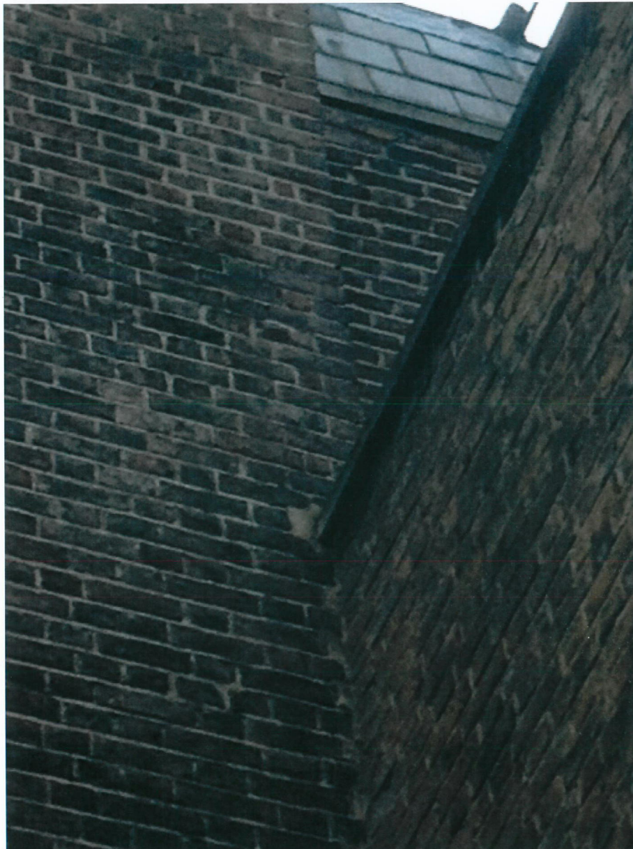
Image 2: detail showing closet wing of 47 Doughty Street overlapping onto the rear elevation of 48 Doughty Street, the Grade I listed home of Charles Dickens.
