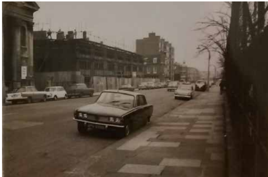
Figure 3.8 View of the former chapel in 1968, with the neighbouring building during construction
