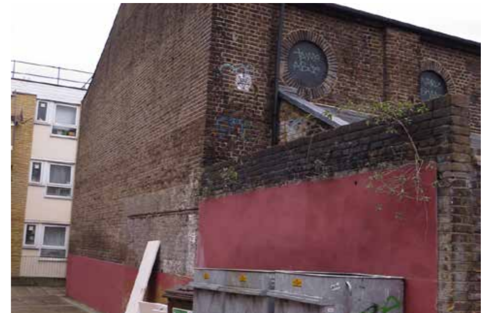
Figure 4.7 View of the rear façade
