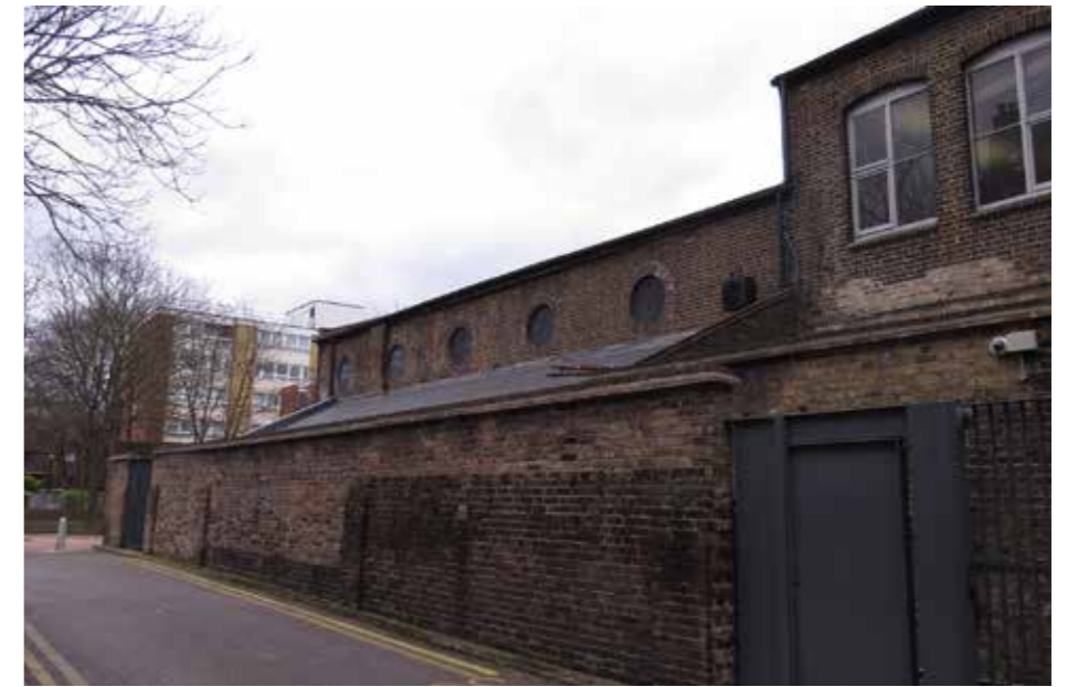
Figure 4.6 View of the west return of the former Methodist Chapel, the rear and middle gallery
