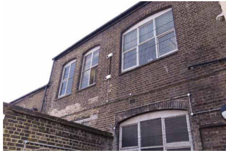
Figure 4.4 View of the exterior of the middle gallery
