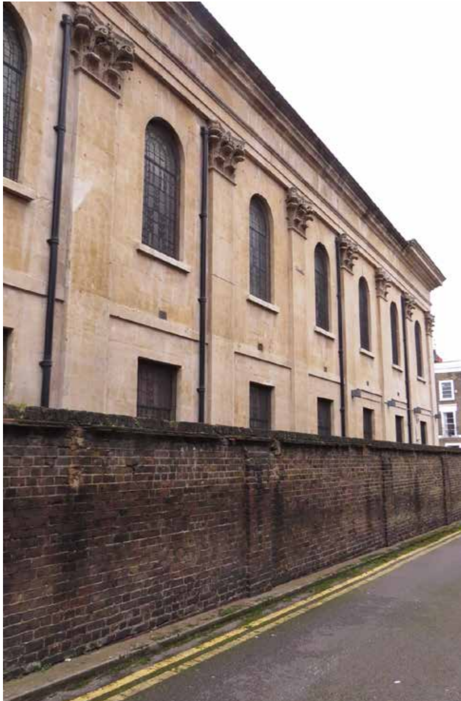
Figure 4.3 View of the west façade of the former Methodist Chapel
