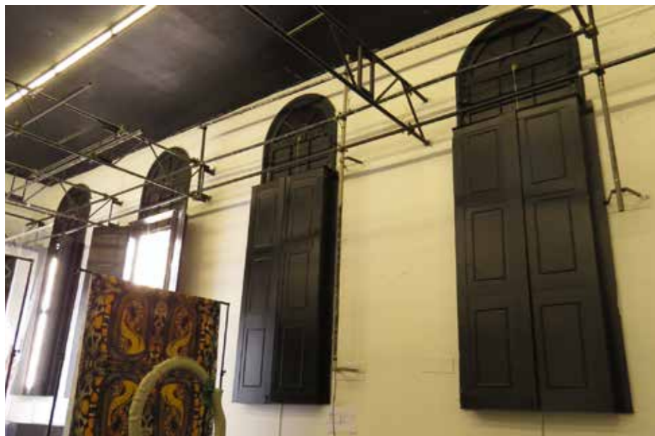
Figure 4.16 View of the rear gallery space
