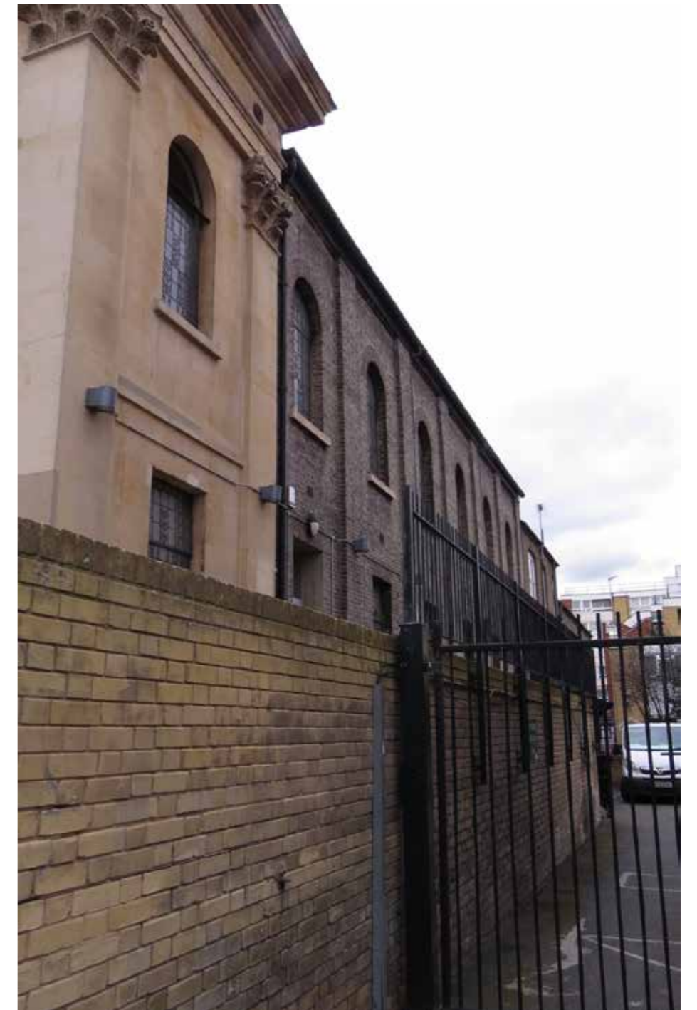
Figure 4.2 View of the east façade of the former Methodist Chapel
