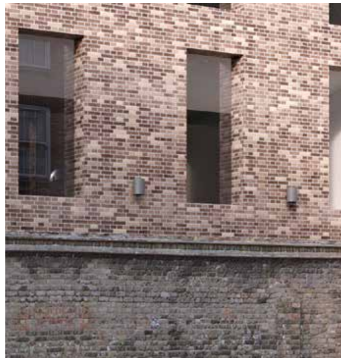
West Elevation - Transition from mixed brick to existing external wall
