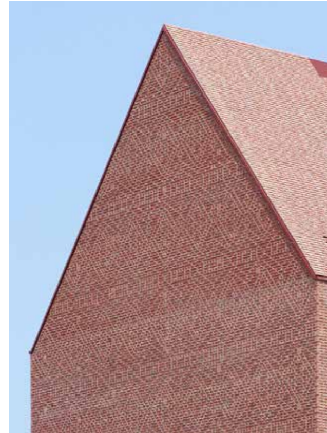
Example of Brick Tiled Roof
