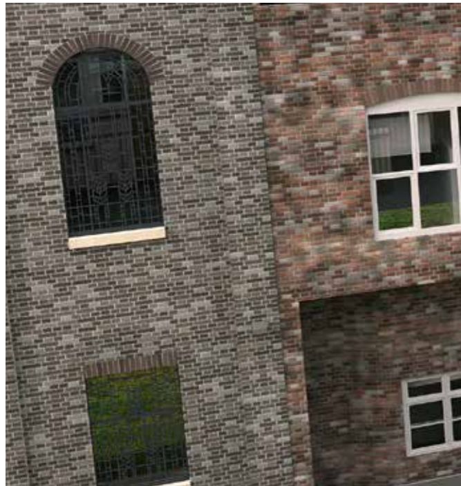
East Elevation - Existing brick transition front to middle galleries
