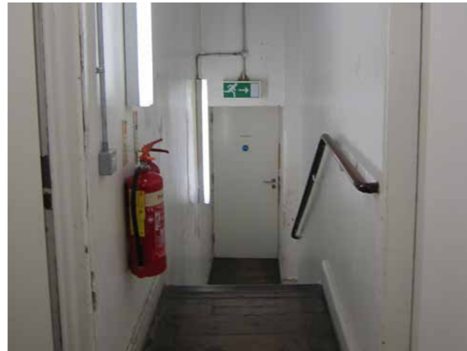
Office - Staircase connecting ground floor and first floor
