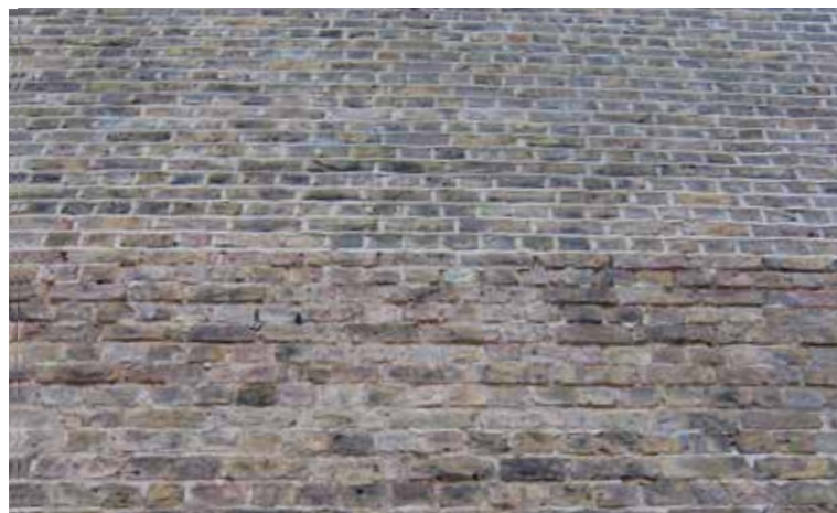
Existing brick to salvage - north elevation
