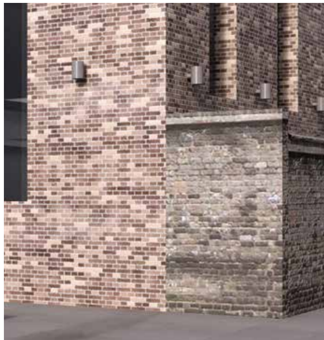
North Elevation - Transition from mixed brick to existing external wall
