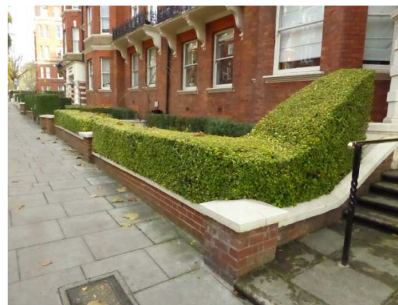
8) Older section of wall, possibly original, which has been reduced in height and capped, following removal of original railings.
