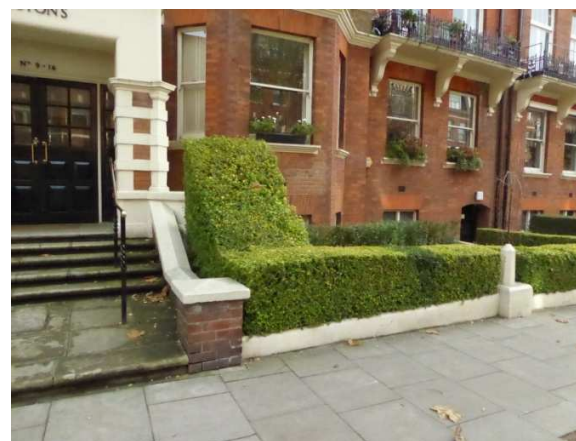
10) Older section of wall, evidently original, which has been reduced in height and rendered. Pier capped with painted stone obelisk.
